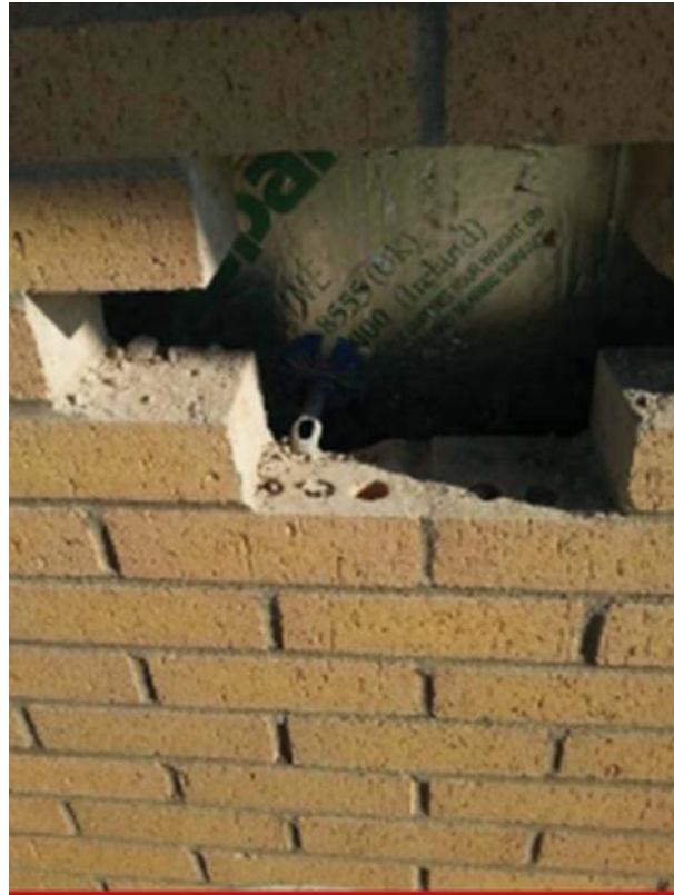
Photo 15.23.45 Location 40 – 35mm embedded
